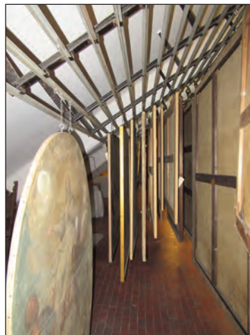
Figure 2 - Palazzo Bianco, Genoa: Sliding painting racks in the attic storage. (Photo M. Loddo, 2017)
