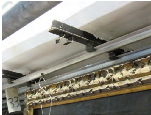
Figure 3 - Palazzo Bianco, Genoa: Hooks connected to rails to hang paintings. (Photo M. Loddo, 2017)
